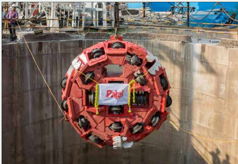
The cutterhead being lowered down the start shaft
