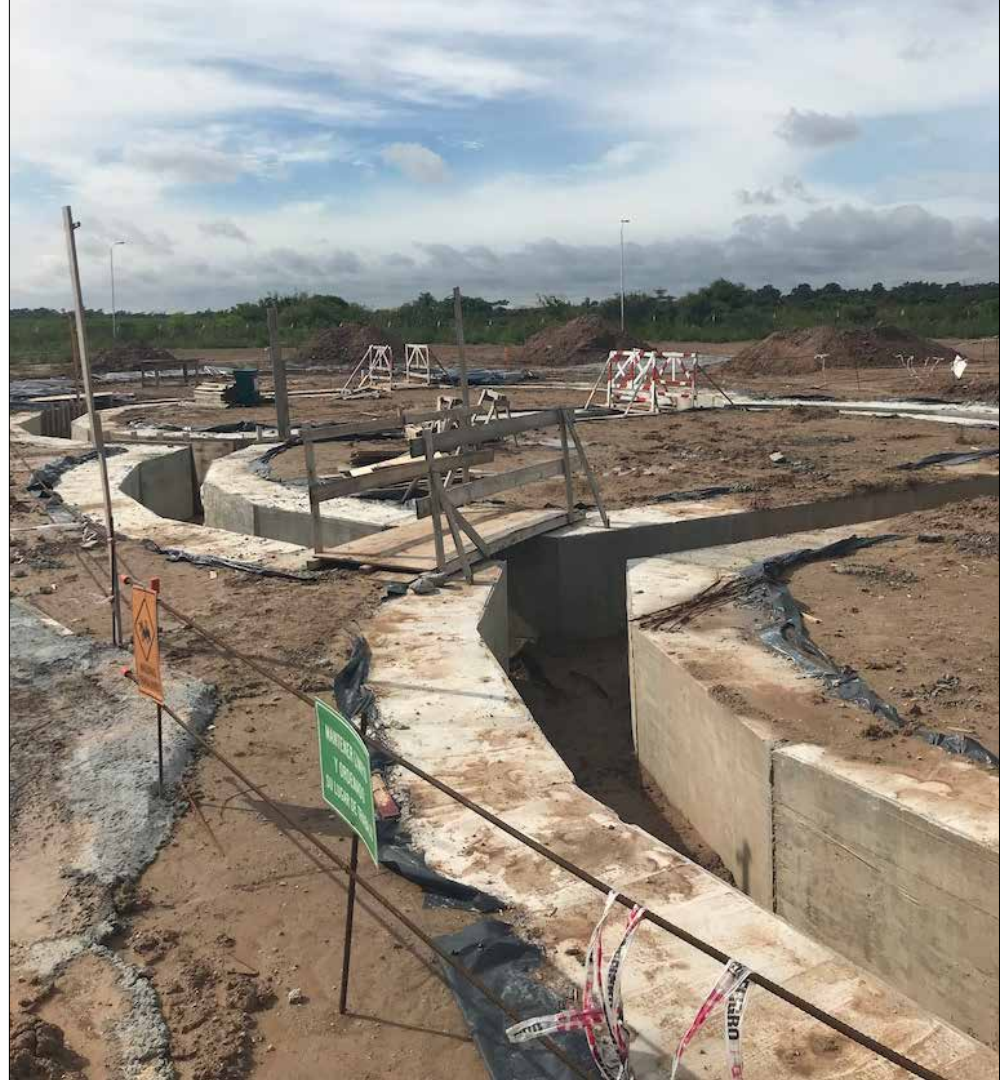
Construction of the four stage launch shaft
