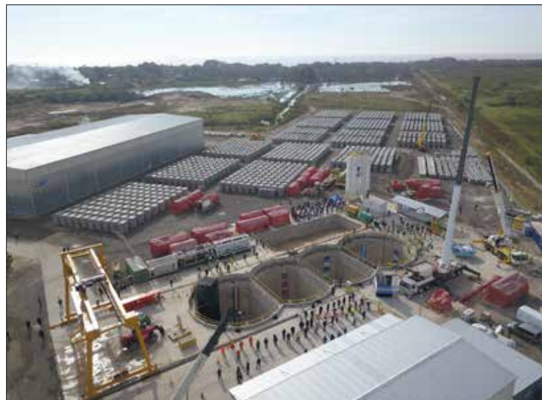
Construction of the four stage launch shaft
