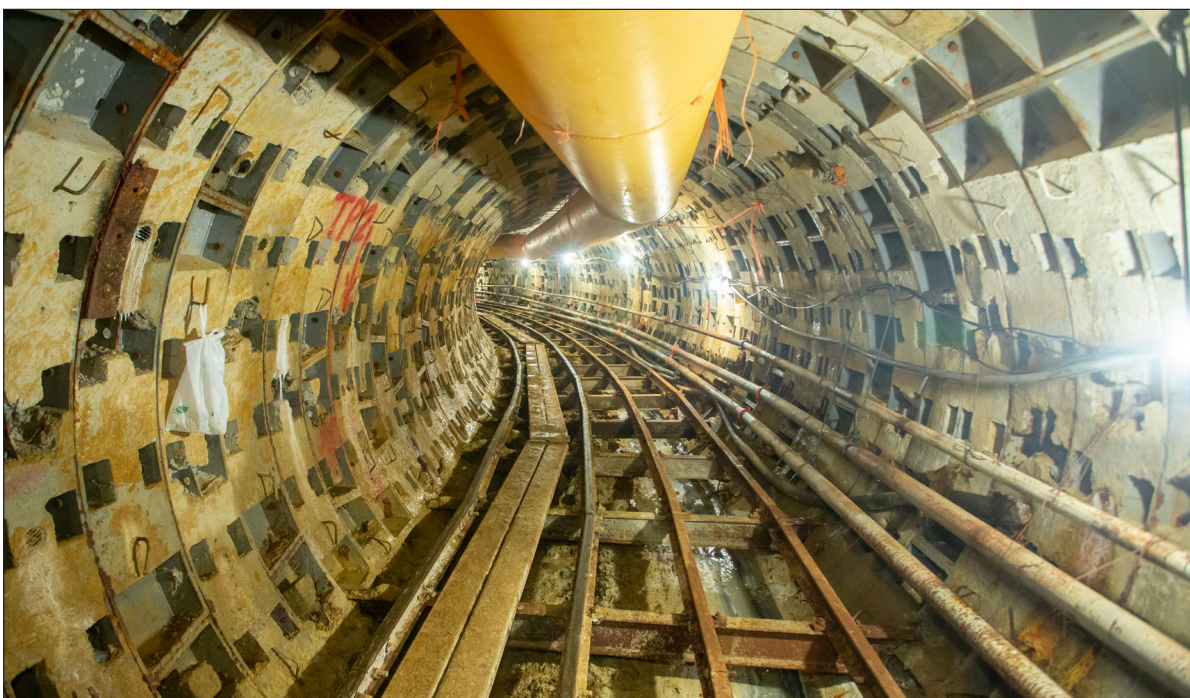
Figure 12. Short steel segment sets in a 35mR curve.
