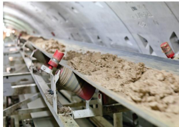
Especially when tunnels are long, when slopes are steep or when space for unloading spoil is limited at the tunnel shaft or portal, the use of a Conveyor System has innumerable advantages over evacuation by rail-bound Muck Cars in terms of productivity, safety and operation and maintenance costs.
