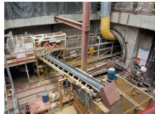
TERRATEC has designed and built sophisticated continuous conveyor systems specifically for individual tunnel and TBM conditions. These include continuous conveyor systems in the tunnel, transfer systems, vertical conveyors and stacker systems at the tunnel portal.
